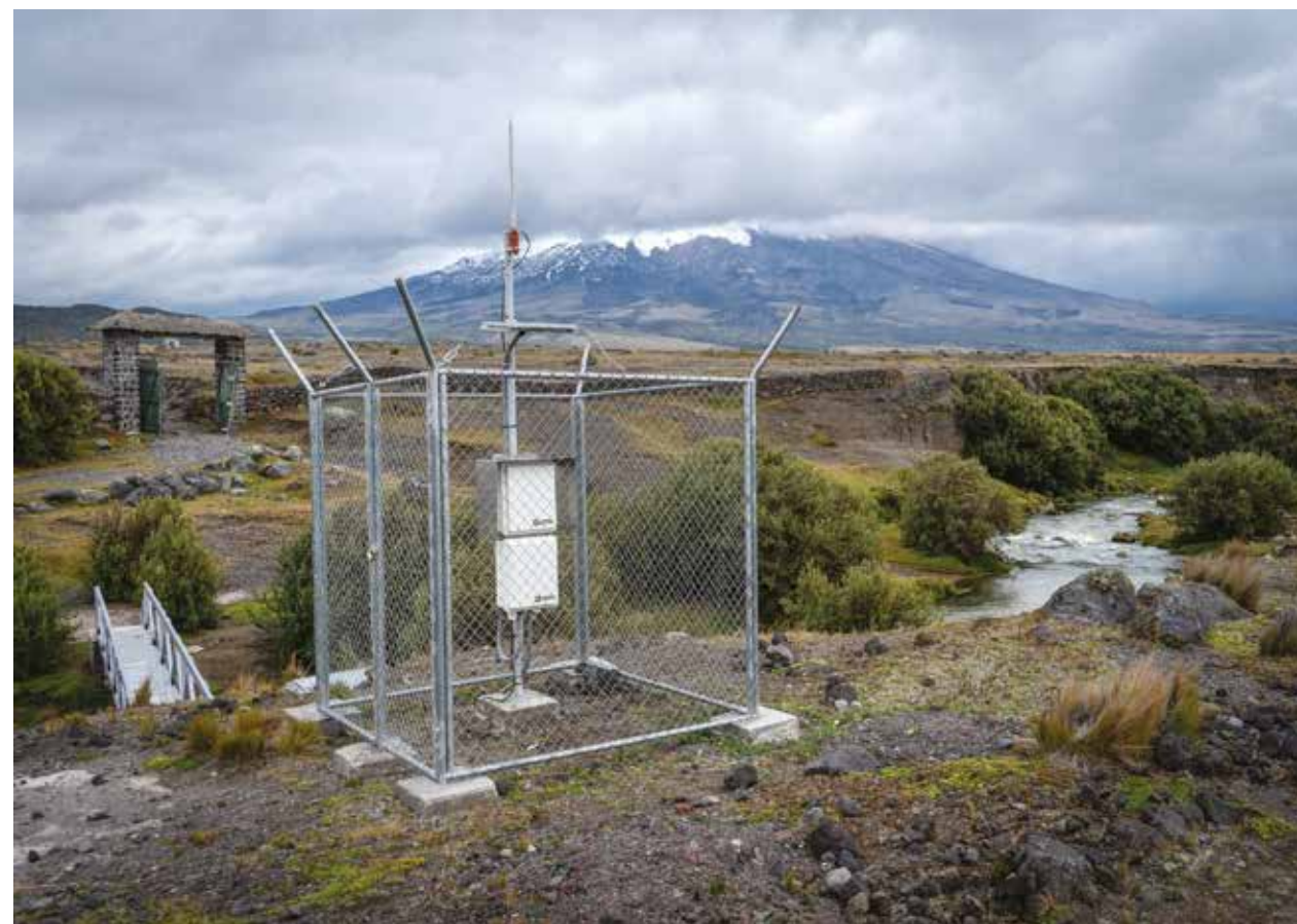
Hydrometeorological Monitoring Station, ACH Alto Pita
